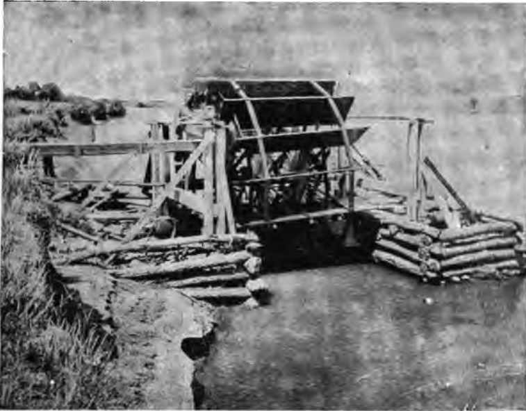
FIG. 19.—Undershot Water-wheel.
